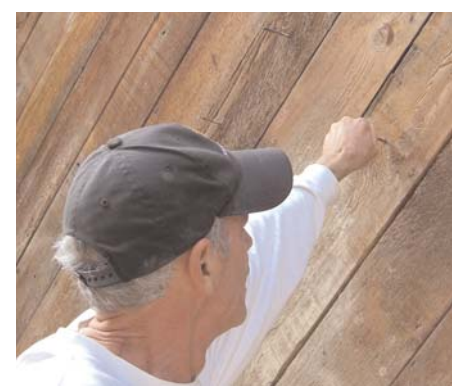
Mike points out one of the old nails that has rusted and collapsed
